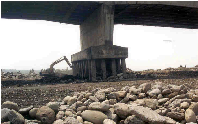
Figure 1. Bed Degradation at Kaoping Bridge, Taiwan causing exposure of pile foundation
