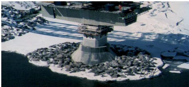
Figure 9 – Armour Stone Scour Pad at Shallow Water Approach Pier (photo by Boily)
