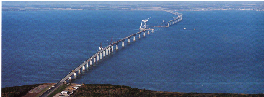
Figure 3 – The Confederation Bridge (photo by Boily)
