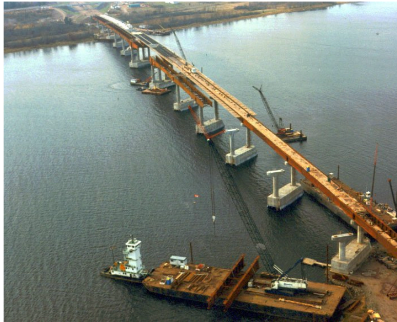
Figure 1 – The St. John River Bridge
