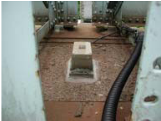
i ) The device on the top of the pier
