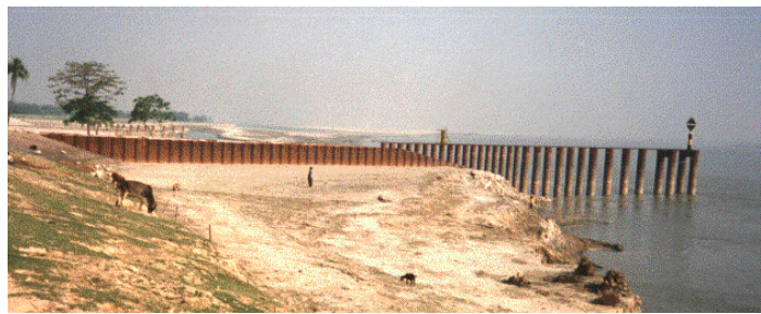
Figure 10 Pile screen as permeable abutment (Jamuna River, Bangladesh).
