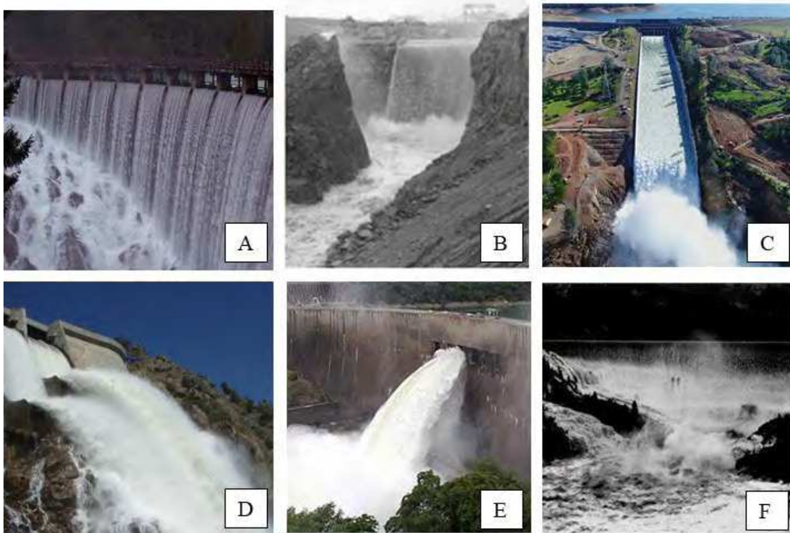
Figure 1. Jet formation due to A) overflow spillway (Lost Creek Dam), B) head-cut formation (Ricobayo Spillway), C) chute spillway (Oroville FCO Spillway), D) flip bucket spillway (Willams Fork Dam), E) gated mid-level outlet (Kariba Dam), and F) dam overtopping (Gibson Dam).
