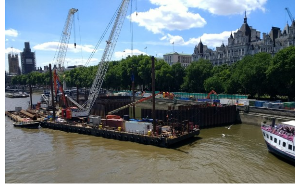
Figure 2. The temporary works under construction at VCTEF.
