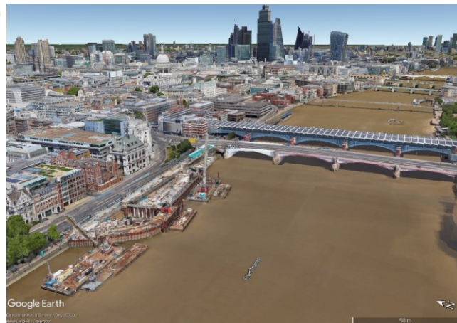
Figure 9. Google Earth image of BLABF temporary works, dated October 2020.
