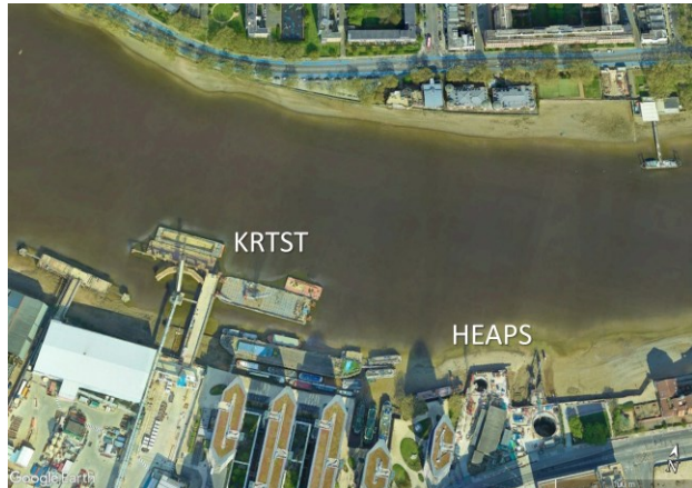
Figure 19. Google Earth image of HEAPS & KRTST temporary works, dated Nov 2020.
