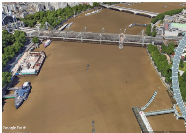
Figure 13. Google Earth image of VCTEF temporary works, dated October 2020.
