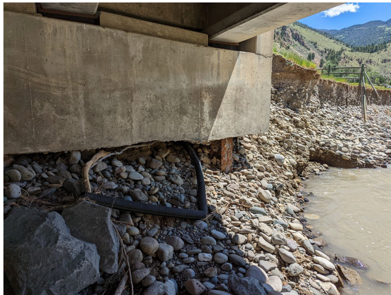
Figure 4. Photograph of upstream corner of northeastern bridge abutment and riverbank.
