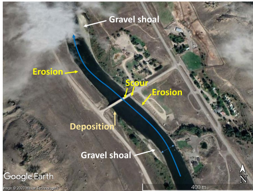
Figure 7. Annotated Google Earth image highlighting erosion and scour hotspots in the context of the river meander and gravel shoals.
