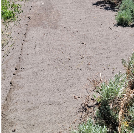
Figure 5. Photograph of sand deposits upstream of the southwestern bridge abutment. Sand ripple wave length was approximately 10 cm.
