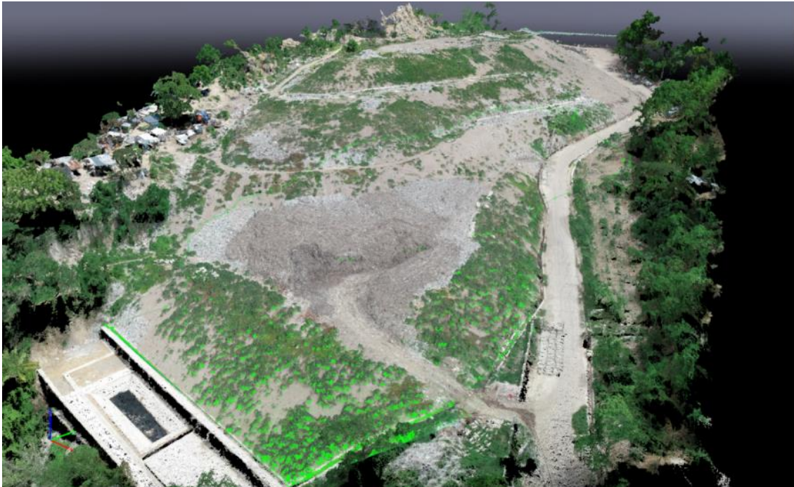
Figure 1. 3D representation of the closed dumpsite based on orthophotos and digital surface model
