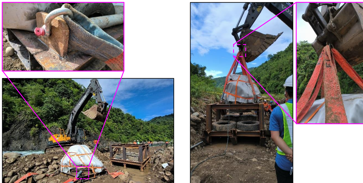
Figure 9. On-site photos during actual lifting (with blow-up images of connections)
