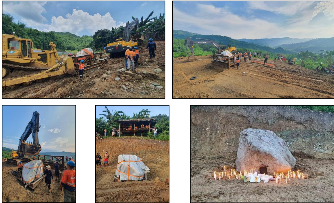
Figure 10. On-site photos during transfer and after unloading
