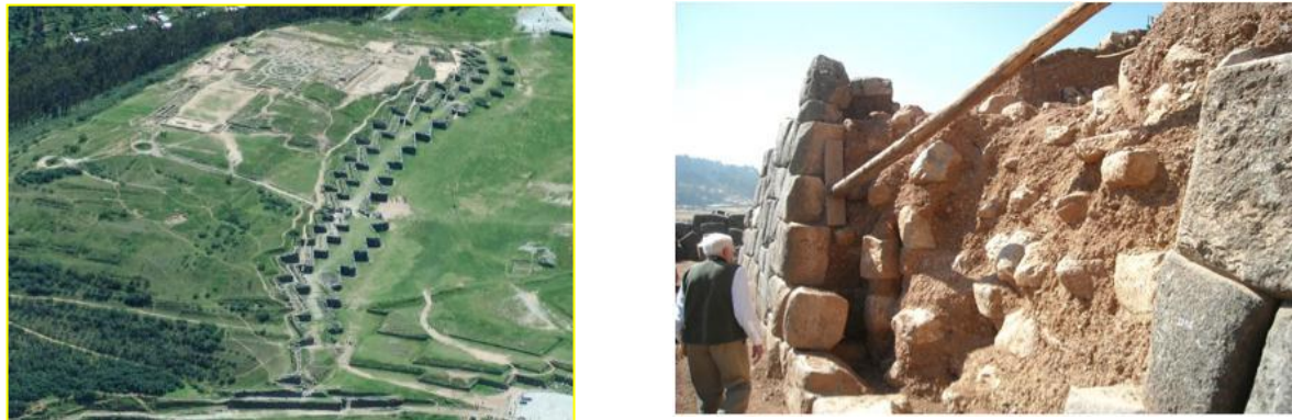
Figure 1. View of Saqsaywaman Park (left). Collapsed Inca wall (right). (Miksad et al., 2013)
