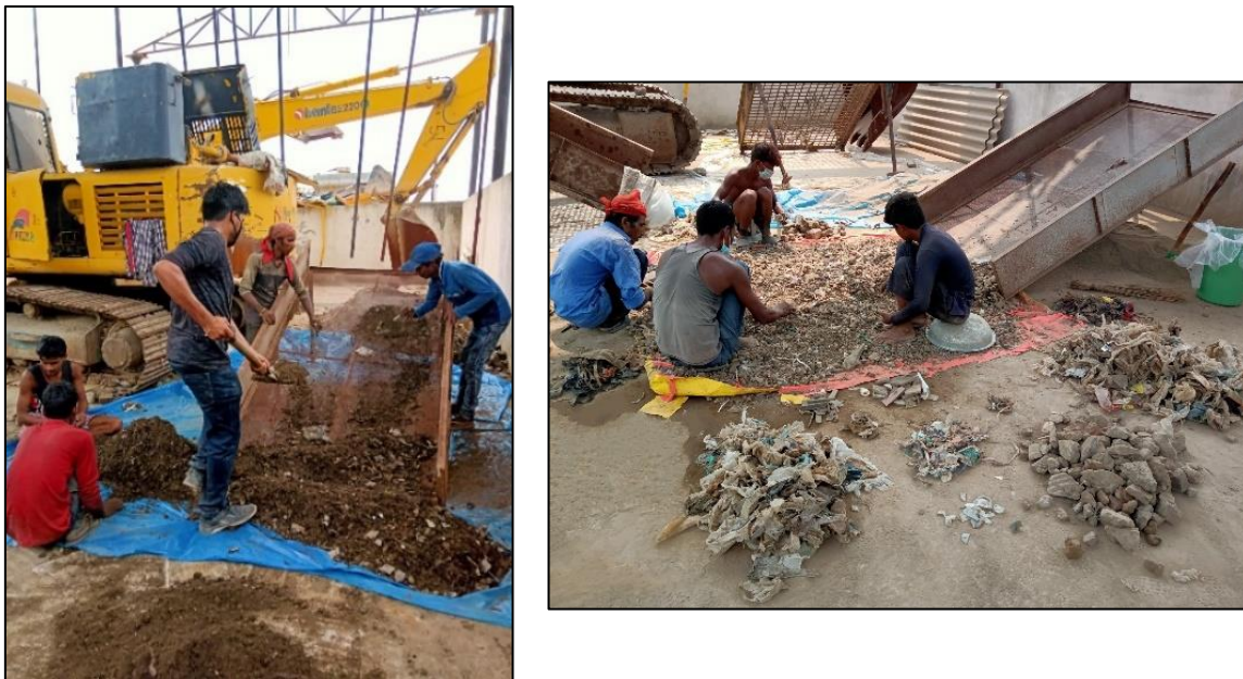
Figure 3. Screening (left) and manual sorting (right) of excavated legacy waste
