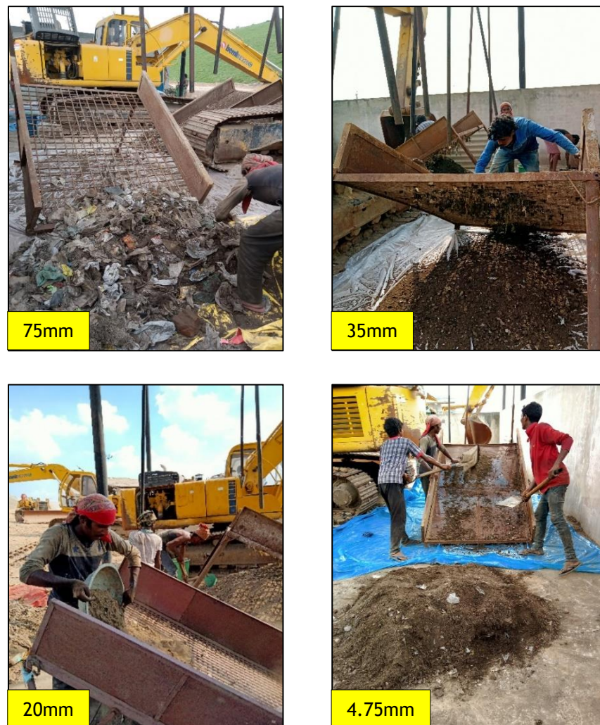
Figure 4. On-site sieving of the dried excavated legacy waste
