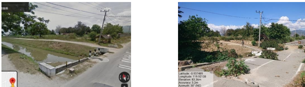
Figure 2. Gumbasa canal at the crest of Petobo slide footprint, before (left) and after (right) the 2018 earthquake (Kusumawardani et al., 2021).
