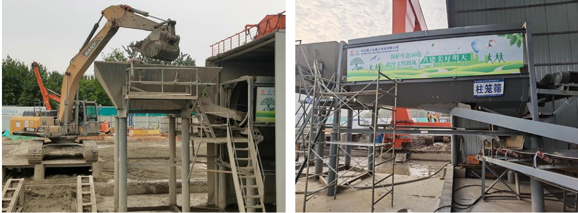
Figure 4. Excavator (left). Cylindrical screen (right)
