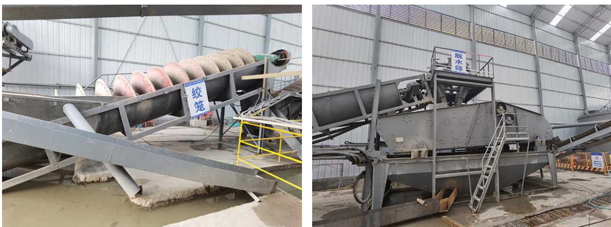
Figure 5. Screw conveyor (left). Dewater screen (right)
