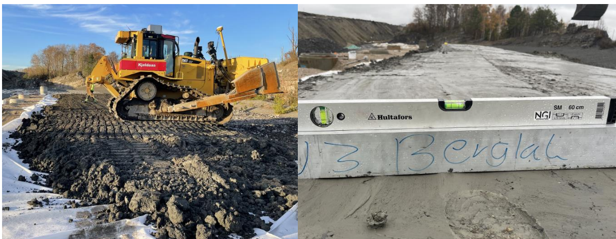
Figure 3. Compaction of the first of three layers (left). Sealing layer surface upon finalization (right).
