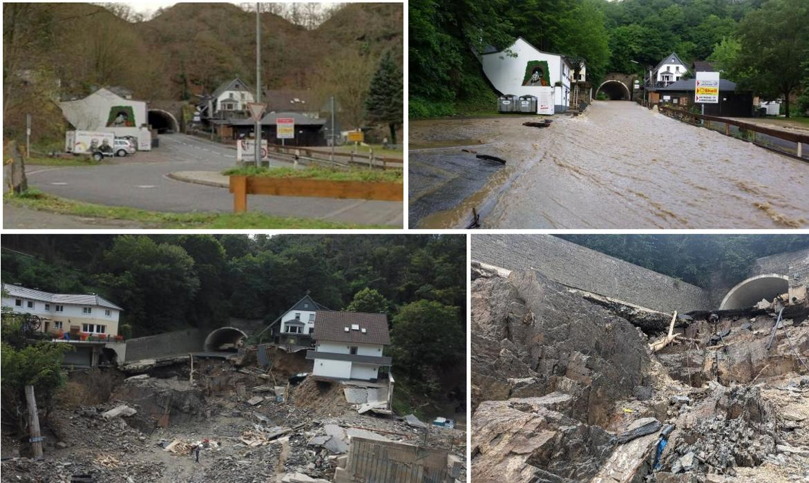
**Figure 8.** Top left: Google Earth/Maps Street View of the Altenahr tunnel from May 2021; top right: photo during the June 2016 flood event (Source: [https://www.altenahr.de/index.php?id=26&publish\[id\]=9709&publish\[mode\]=overview&no\\_cache=1#18](https://www.altenahr.de/index.php?id=26&publish[id]=9709&publish[mode]=overview&no_cache=1#18)); bottom: photos by the reconnaissance team after the 2021 flood, August 2021 (50.5165261, 6.9975355)
