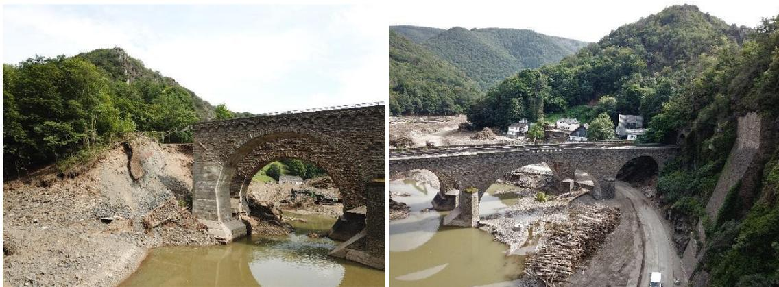
**Figure 12:** Photo of the abutment region of the double bridge, August 13<sup>th</sup>, 2021. Left: Washed out abutment area, Right: bridge abutment area intact and connected to adjacent rock slope
