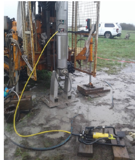
Figure 8. Insertion of bottom sealing cap
