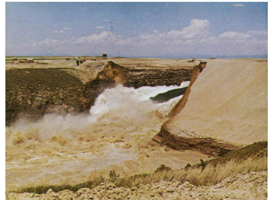
Figure 1. Teton dam was destroyed (Independent panel to review the cause of Teton dam failure 1976).
