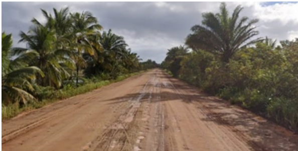
Figure 3. Frontal view of the region where the test section will be implemented on the BR-030/BA highway
