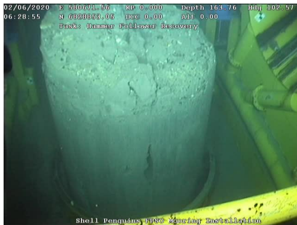
Figure 3. Pile plug sticking out of the pile as seen from the piling template after removal of the follower.
