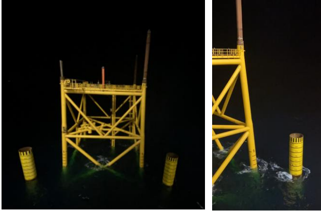
Figure 9. The first batch of two stabbed piles and a close view of one of the piles during pile movement monitoring.
