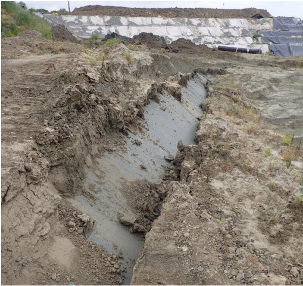
Figure 4. Observed shear failure on a pre-existing failure plane in the clay pit at Rumbeke (image credit: Jan Maertens)
