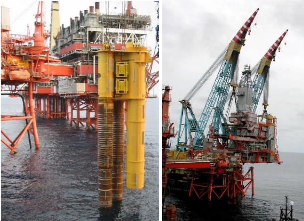
Figure 52 The piggyback repair system (from Alm et al., 2004) and IP jacket topside installation
