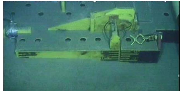
Figure 17 Example of uneven shallow foundation skirt partial penetration due to the presence of drill cuttings.
