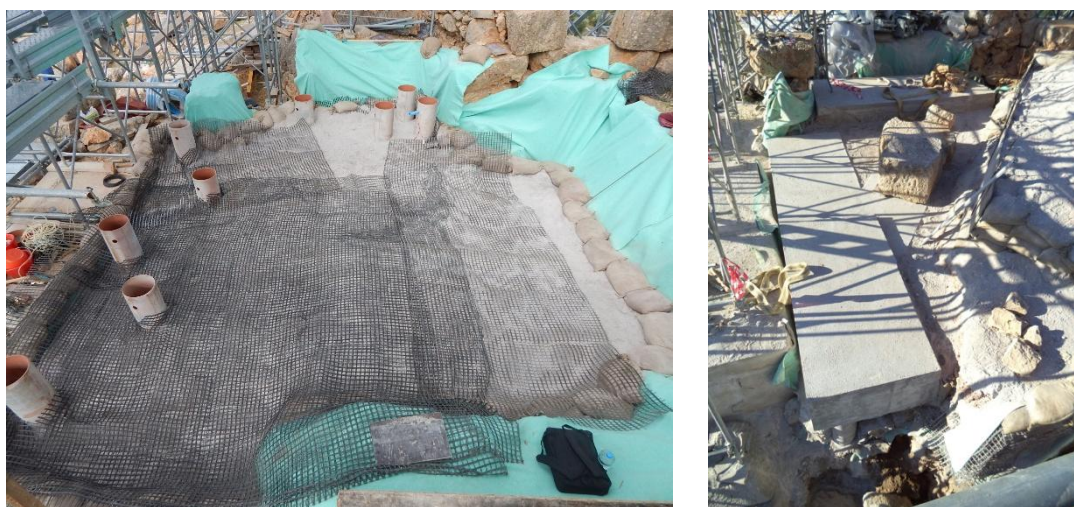
Figure 11. The deep foundation under construction (view from the east) (left). The pile cap of the eastern elevation before the anastylosis and, in the background the western one (right).
