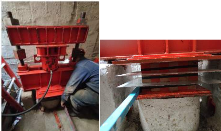
Figure 10. Load application at 90 t. Pile 54/205B.
