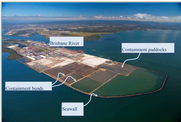
Fig. 1 Aerial view of land reclamation site at Port of Brisbane, Queensland, Australia
