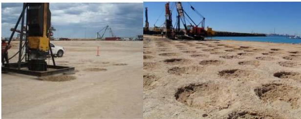
Fig. 3 CDYC dynamic compaction in operation
