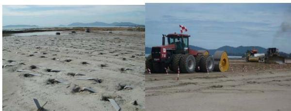
Fig. 5 PVDs and HIEDYC compaction used for dynamic consolidation
