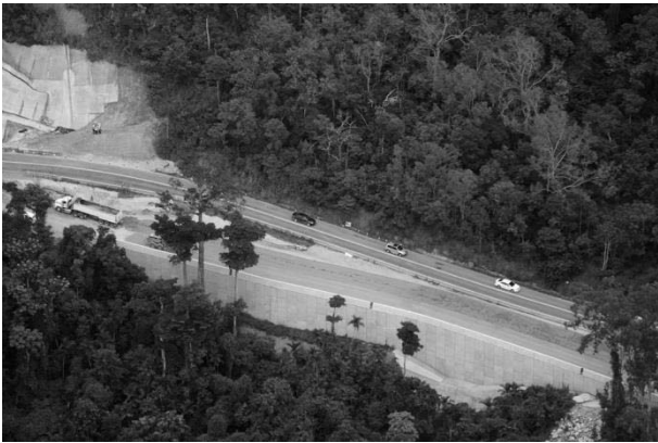
Fig. 2 Setting of SMSE Wall (photograph taken near end of construction)
