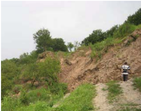
Fig. 6, new landslide on June 7, 2009
