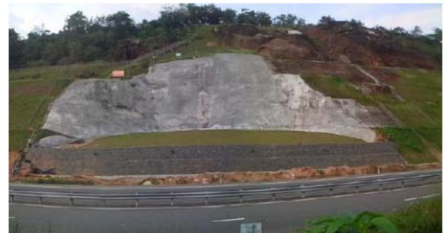
Fig. 12 Slope after completion of rectification
