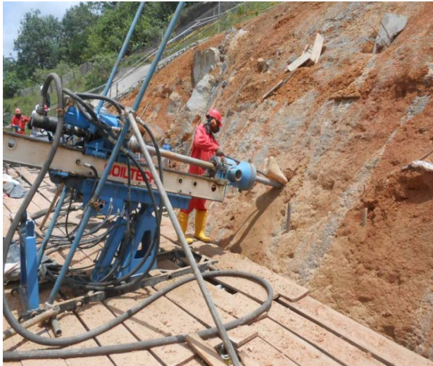
Fig. 7 Drilling for soil nailing /cable anchoring
