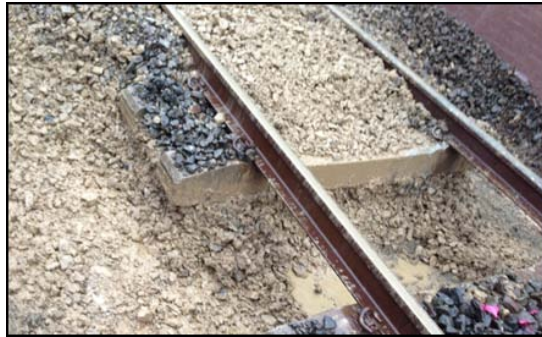
Fig. 2 Ballast fouling due to clay pumping (Photograph were taken during track maintenance at Ashfield, NSW).
