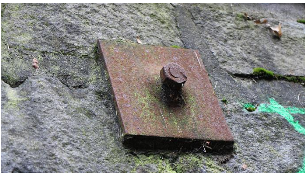
Figure 4. Short-headed tendon face on legacy anchor
