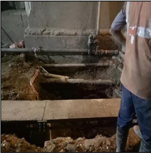
Figure 12. Photograph of placing of ramp.
