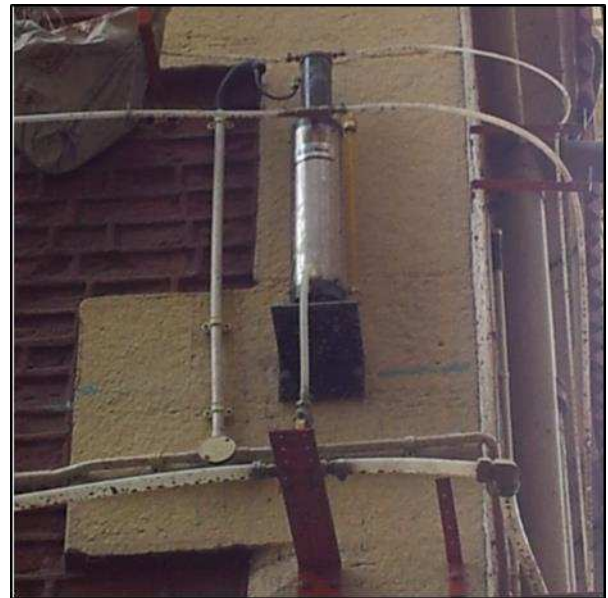
Figure 6. Photograph of settlement sensor.
