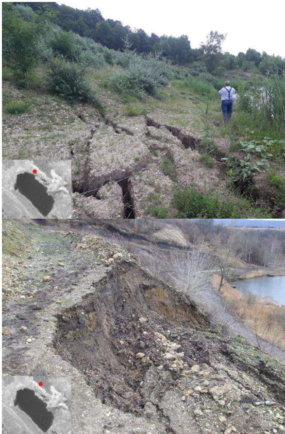
Figure 2. Surface cracks and landslide on the slope NE to the lake. (Red dot indicates point of view of the photos)
