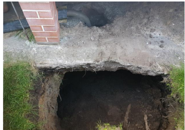
Figure 2. Typical surface expression of pothole subsidence of shallow mine workings, and filling with concrete.
