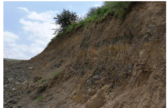
Figure 6. Outcrop of weathered clayey marl
