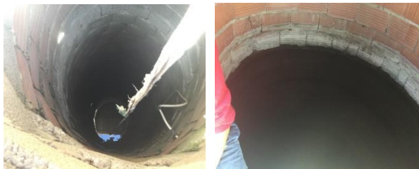
Figure 7. Several wells located in the sliding zone
