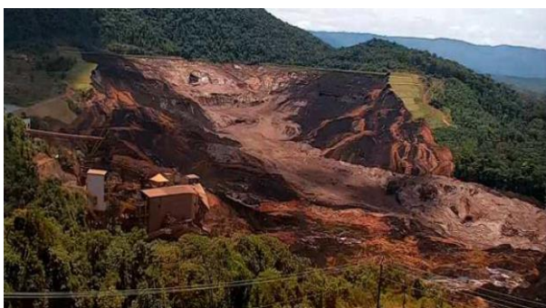
b) 6 min. after the first observed deformation Figure 1. Brumadinho Dam failure (Robertson et al., 2019).
