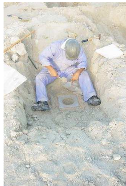
Figure 6. Execution of a sand replacement test.
