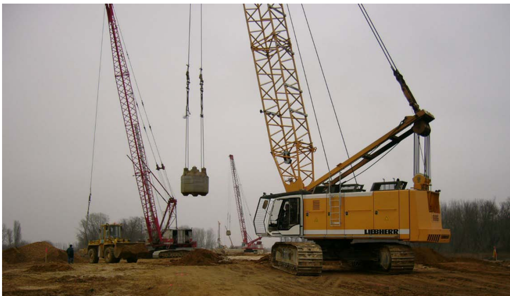
Figure 4. Application of dynamic replacement in the project.
