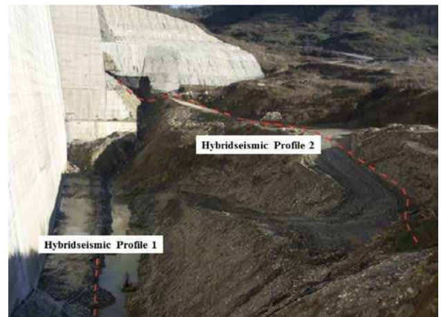
Figure 11. Case study 1: Dam site with position of two authentic hybrid seismic profiles
