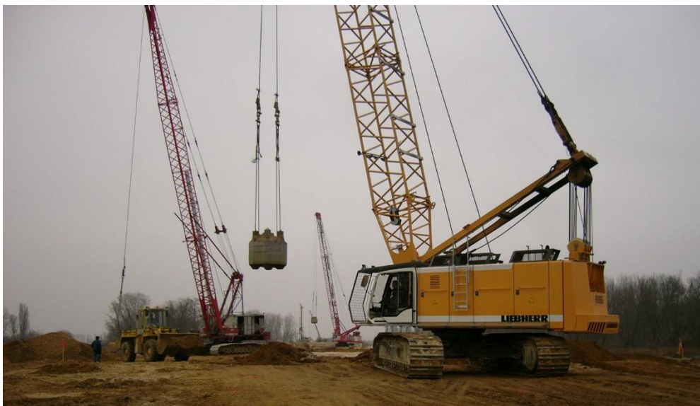
Figure 4. Application of dynamic replacement in the project.
