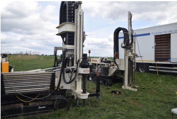
Figure 2. Application of two DP machines for CPT-based seismic tomographic measurements.
