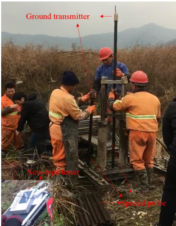
Figure 10. Field Tests of Wireless Static Penetration System
