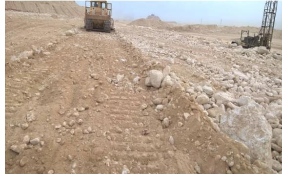
Figure 15. Spreading of rock fill material.
