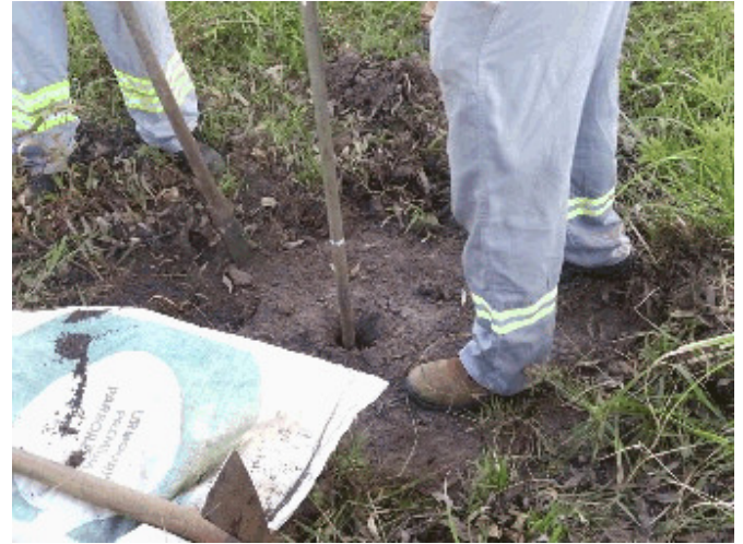
Figure 6. Sampling auger for geotechnical characterization of materials
