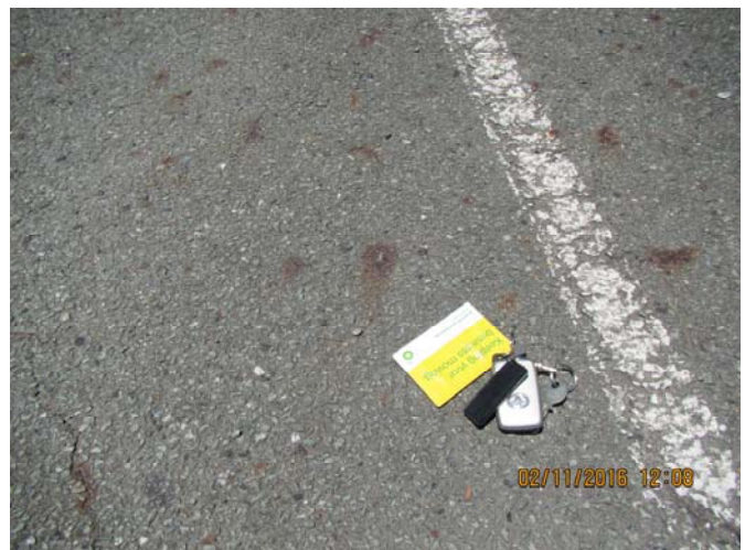
en colour pyrite ( \text{FeS}_2 ). Aerial oxidation of pyrite could result in adverse discoloration in aesthetic concrete & road surfaces. Figure 5. An example of aerial oxidation of pyrite ( \text{FeS}_2 ) bearing asphalt aggregate on a road surface showing scattered and spotted rusty red brown discoloration.
