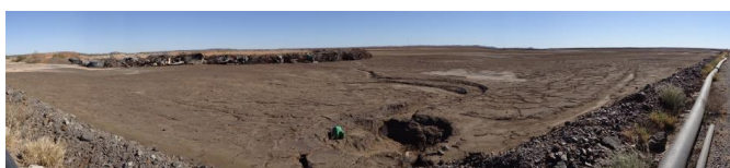
Figure 2. View of heavily desiccated surface of Cannington's surface TSF Cell 1.
