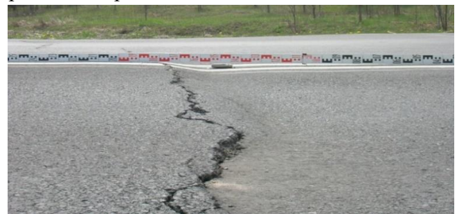
Pic. 2-1. A linear-type discontinuous surface deformation (Grygierek 2010)
