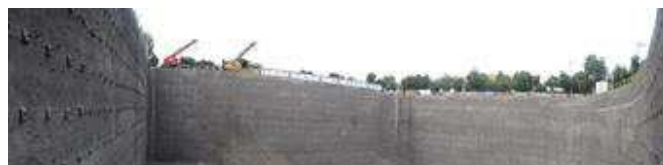
Fig. 1 A view of walls stabilized by nailing
