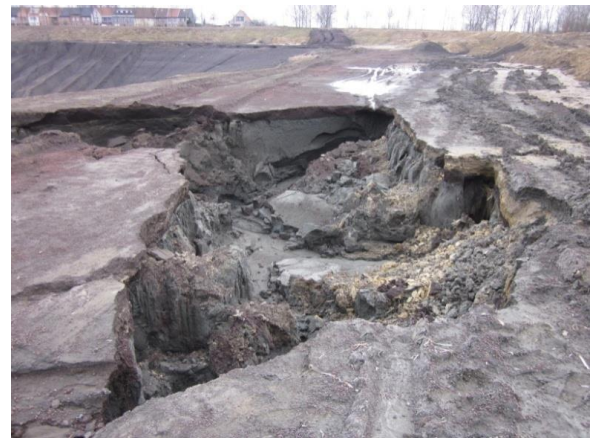
Figure 3. Detailed impression of the instable slope
