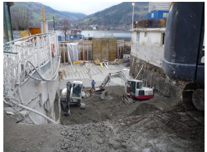
Figure 9. Picture of excavation and soilcrete columns
