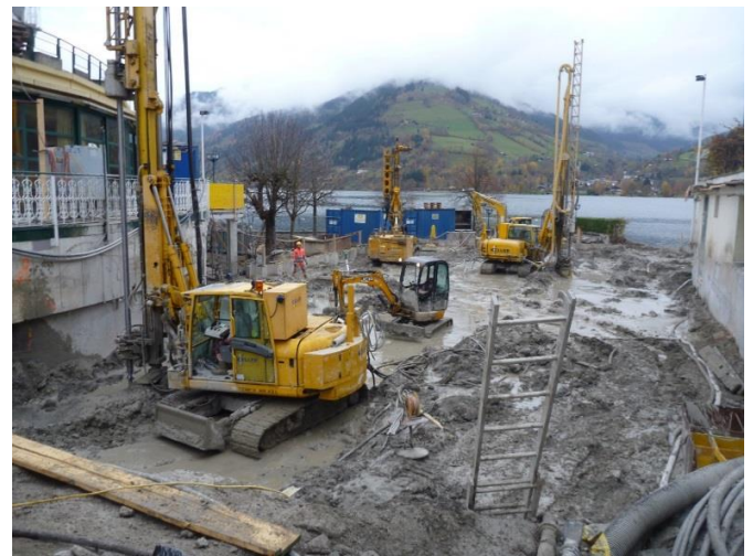
Figure 8. Picture of Jet-Grouting-Works
